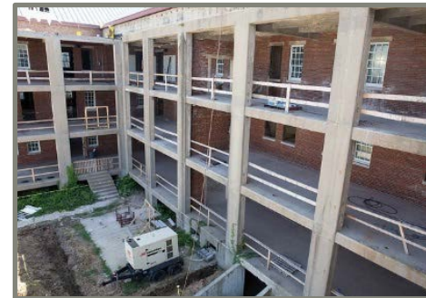
Hale Hall Renovation Fort Meade, MD
