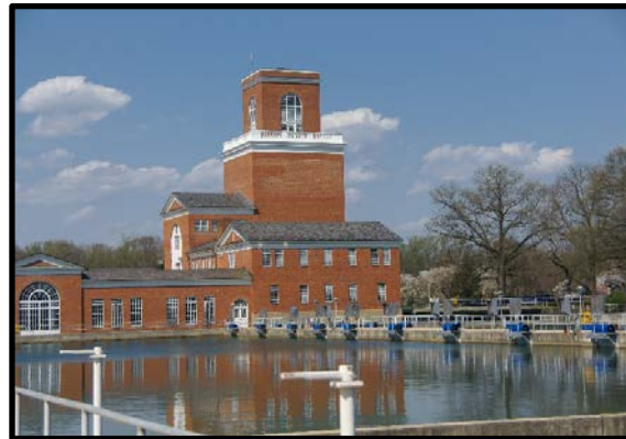
Dalecarlia Water Treatment Plant
